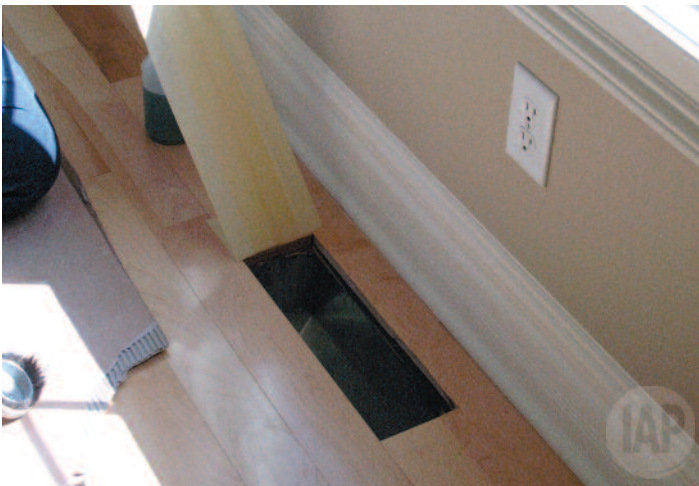
All sealing is carefully removed from registers in each room.
