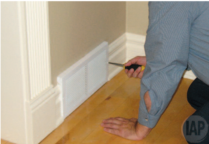
All register covers are carefully replaced.
