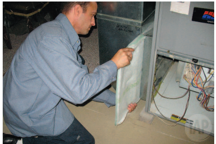
We install a new, high performance furnace filter featuring an antimicrobial coating.
