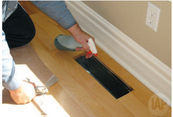
Register boots are then wiped down.
