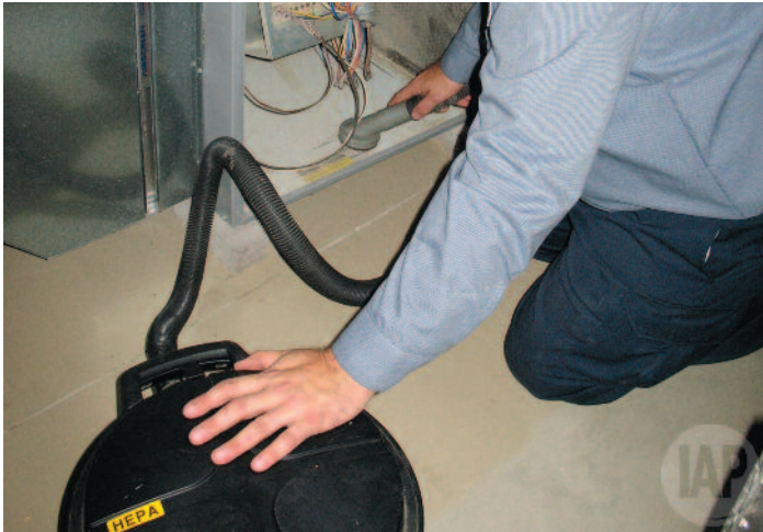
Furnace blower section is thoroughly HEPA vacuumed and cleaned.
