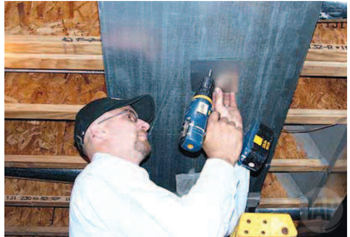
Access holes are sealed with silicone caulked plates and screws for an air-tight finish. Plates can be easily removed for your next duct cleaning.
