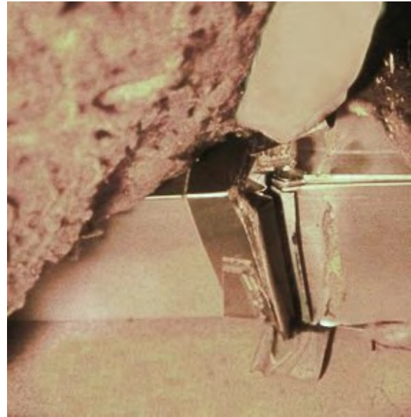
Figure 3. Failed duct tape on this joint under attic insulation could have gone undetected for the life of the home.
