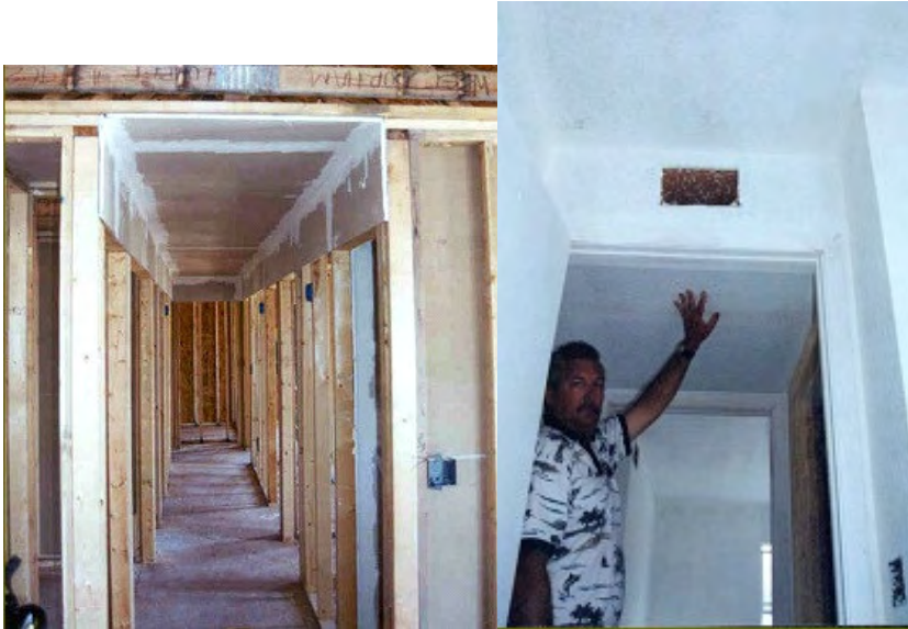
Figure 17. Duct chase installed in an 8-foot hallway. Note finished system is just above door trim.
