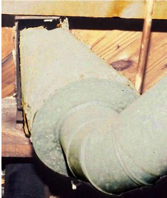
Figure 2. Ducts disconnected from boots are surprisingly common. Mastic with imbedded fiberglass results in a strong, long-lasting repair.
