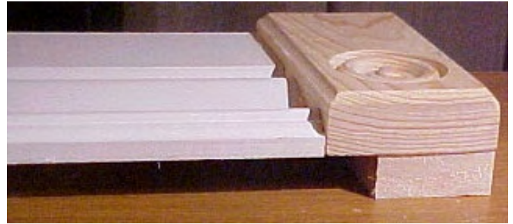
Figure 18. The deKieffer Bypass uses the space between an interior door's header and the beginning of drywall above the door which starts at the height of the trim. The trim on top of the doorway is offset to allow flow. A sheet metal scoop attaches to the drywall on both sides of the opening to provide integrity.
