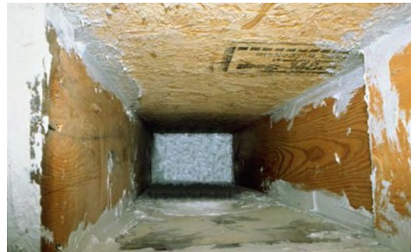
Figure 4. Panned duct repair needs to be thorough, not necessarily aesthetically pleasing.
