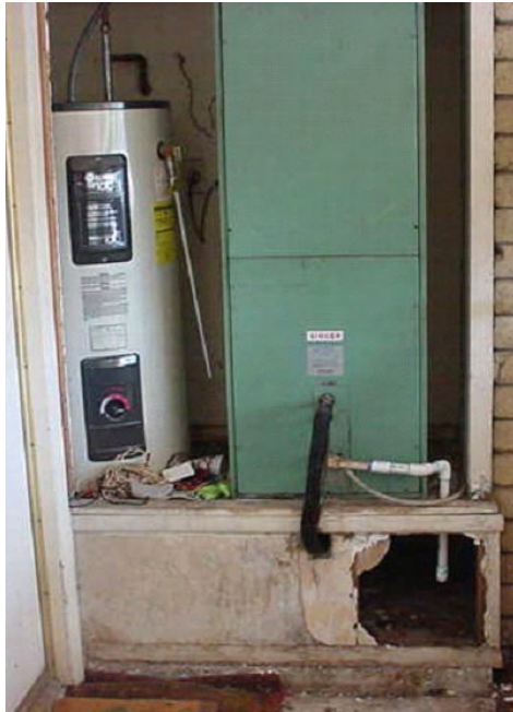
Figures 5 (before) and 6 (after). Air handler mounted on a platform in an unconditioned garage.
